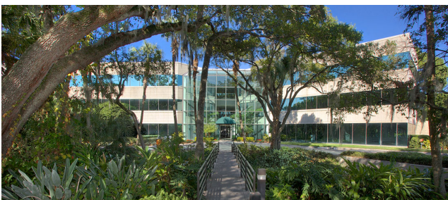
CYPRESS CENTER III 5405 CYPRESS CENTER DR. | TAMPA, FL 33609
